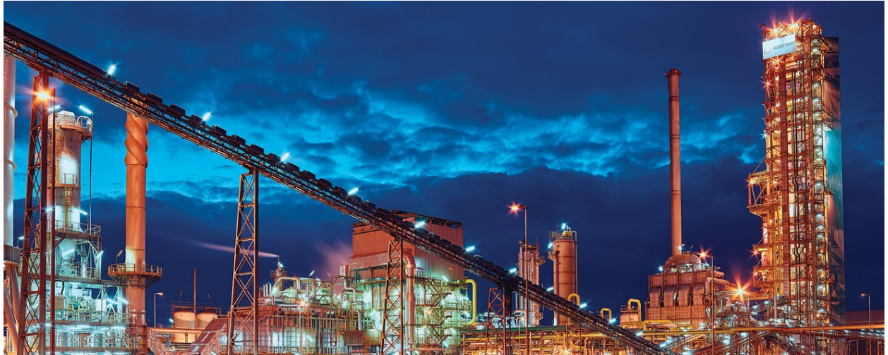
© Ezz Steel Company – Alexandria (EZDK)
